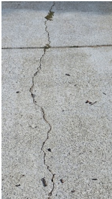
Sidewalk Material Concrete.
